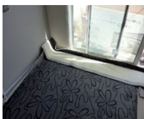
Implantation de la moquette Laying the carpet
